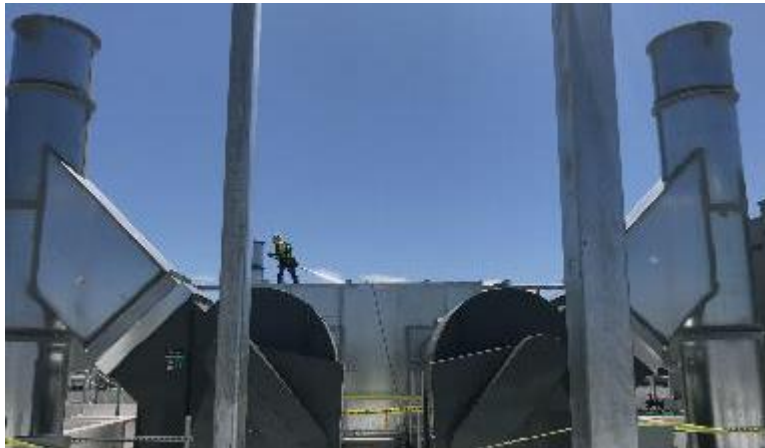
Roof Level Building Exhaust Stacks
