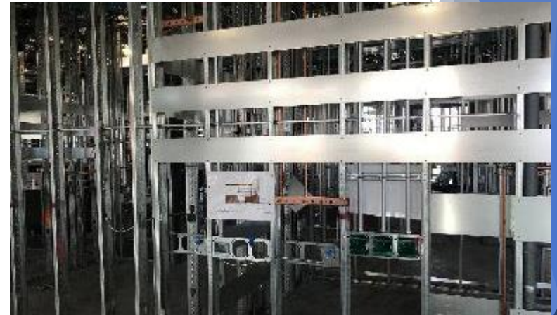
4 th Floor Inwall Utilities & Mounting Support
