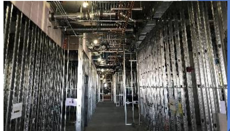
4 th Floor Wall Framing & Overhead Utilities
