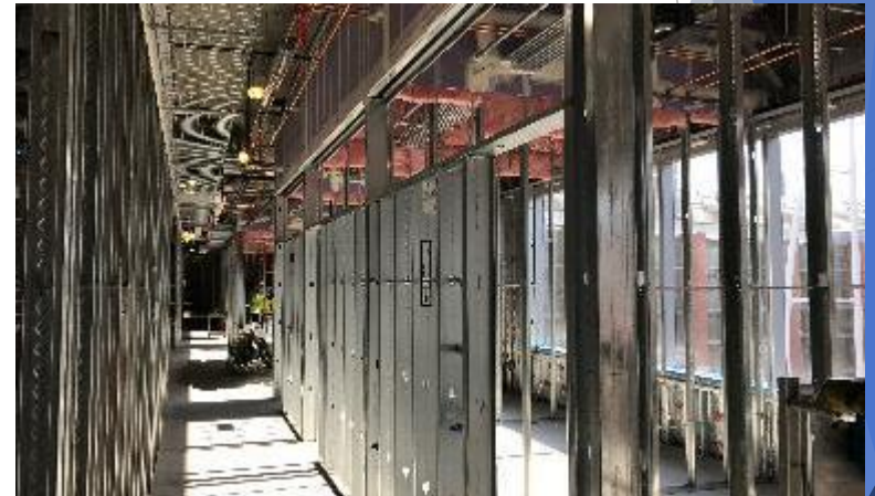
4 th Floor Wall Framing at Perimeter Rooms
